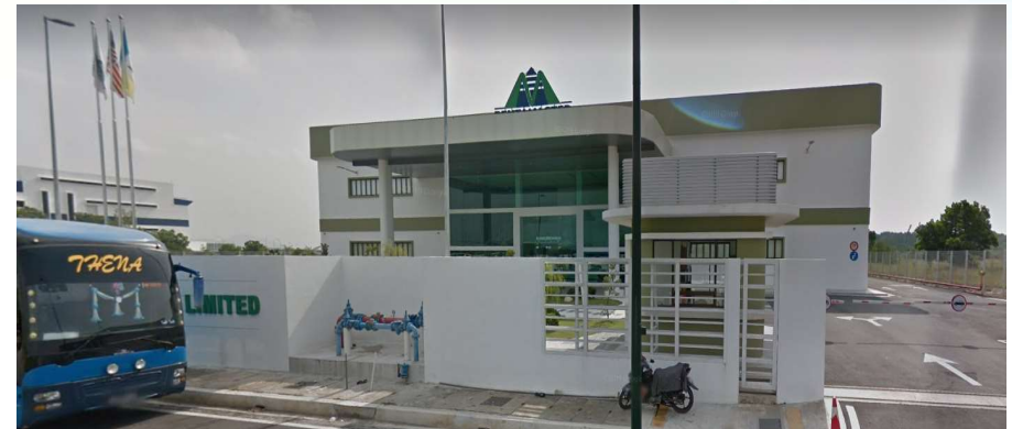
Second plant located at Batu Kawan, Penang, Malaysia.
