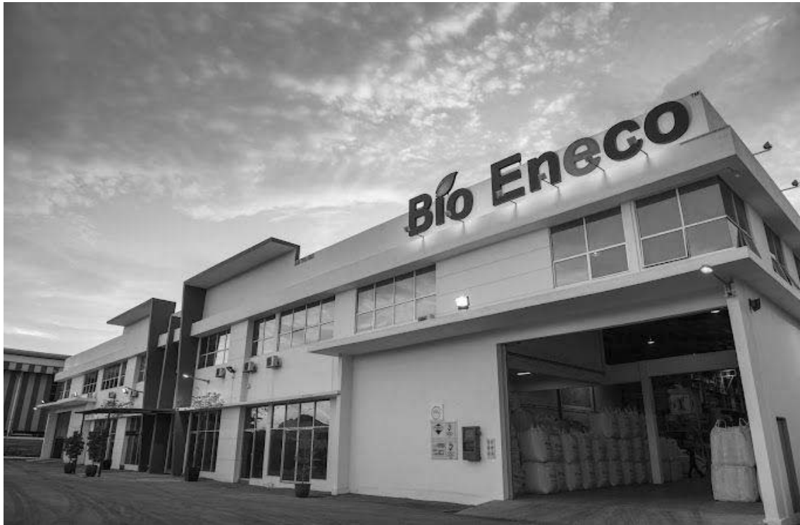
Entrance of Port Klang Factory
