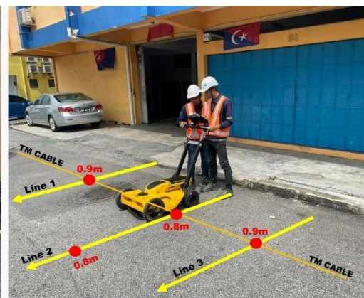
Tracing officers detecting the underground utilities using GPR
