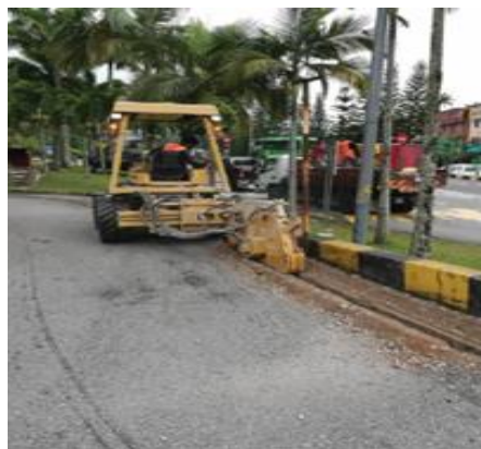
Our micro trencher being operated at a project site
