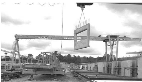
Removal of formwork (i.e. IBS component) for storage
