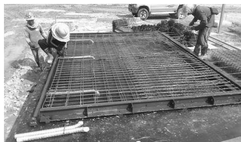
Assembly of framework within the formwork
