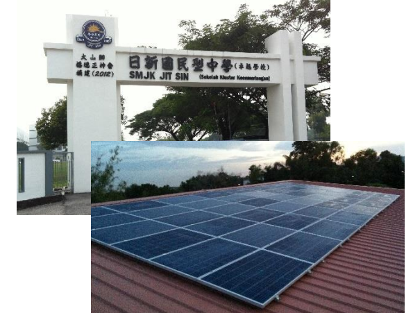
48kWp solar PV system for SMJK Jit Sin with O&M
