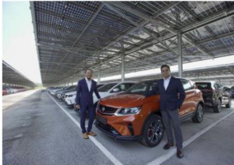
Pekát Group Bhd executive director Wee Chek Aik (left) and Proton Holdings Bhd investment and promotion director Mohd Khalid Yusof at Proton Holdings Bhd's Tanjung Malim plant, Perak. Pekát Holdings Bhd completed a RM33.1mil, 12 megawatt-peak grid-connected solar photovoltaic system at the plant.
