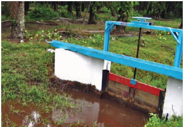
Weir to control water level in canal
