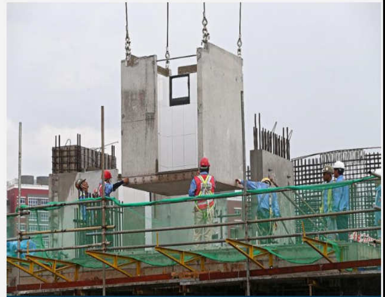
Prefabricated bathrooms units are assembled with finishes in a factory before it is transported to a construction site for installation. PHOTO: LIANHE ZAOBAO
