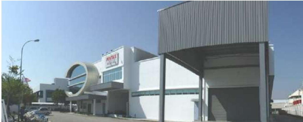
1. Bayan Lepas Industrial Facility 1, Penang
