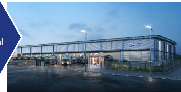
Skylights and Energy-efficient lighting
