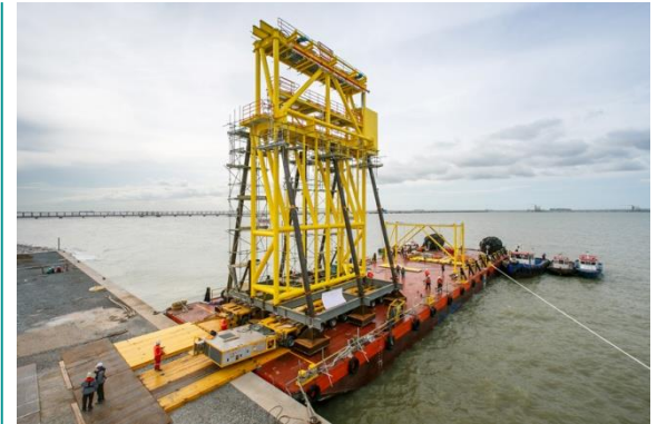
Heavy Engineering Fabrication (Offshore)
