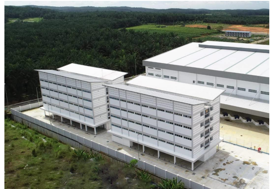
2 BLOCKS OF HOSTEL FOR STAFF SCGM INVESTED RM8 MILLION IN 2018/2019 TO UPGRADE ITS STAFF QUARTERS.
