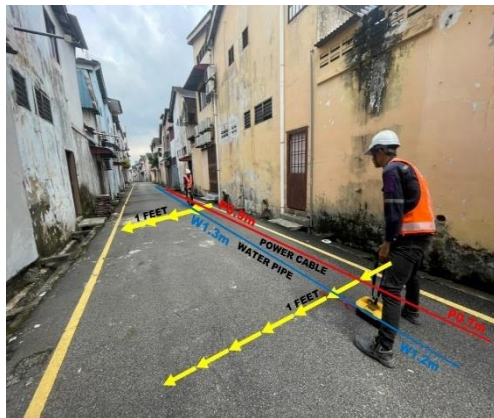
Tracing officers identifying the number of utilities present underground using induction method of PCL
