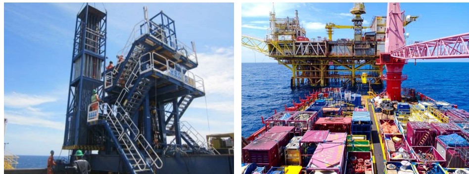
Pulau A IWS Well Equipment and Marine Spread
